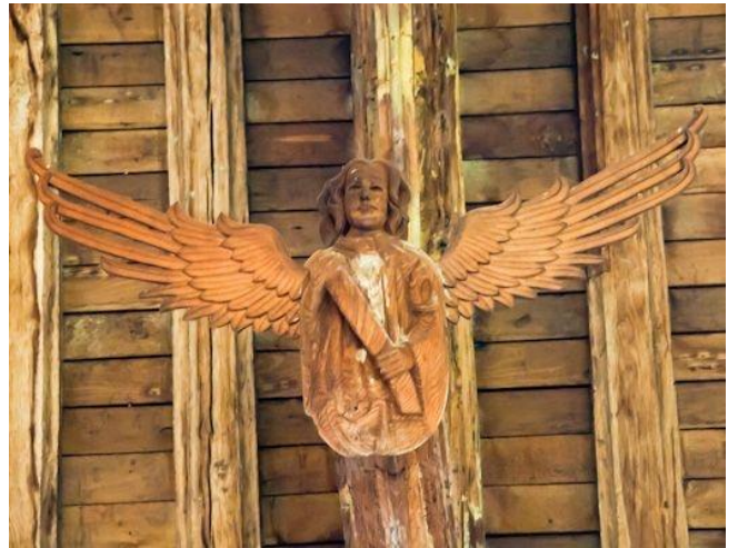
An example of an Angel repaired by Henry Brett's men.
