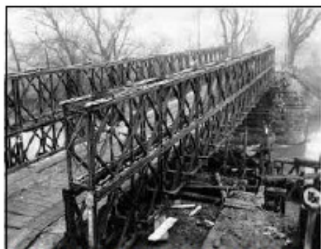
A Bailey Bridge but not at Stanton
